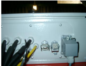
Plug from the remote connected on the control panel
